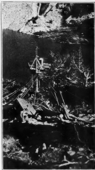
Above, Buckets Landing on Rails; Below, Method of Anchoring Cableway
